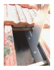
3.Remove tiles where the rafter is and bolt on the bracket (make sure the top extruding from roof is 90 degrees. Repeat this process with all the brackets.
