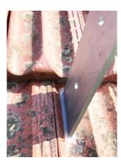
4.Mark where the bracket will protrude through the tile and then use a grinder/tile cutter to cut a slot to size. Replace the tile and Sikaflex around the bracket. Make sure it's waterproof.
