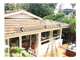
6. Add a timber beam to the width of the awning. The beam required is 180mm x 50mm. Paint with outdoor timber paint to your desired colour scheme. Add the brackets from the COCOON awning. Adjust the pitch to match on each.
